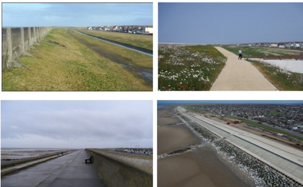
Figure 13: Rossall Coastal Defences Before & After
